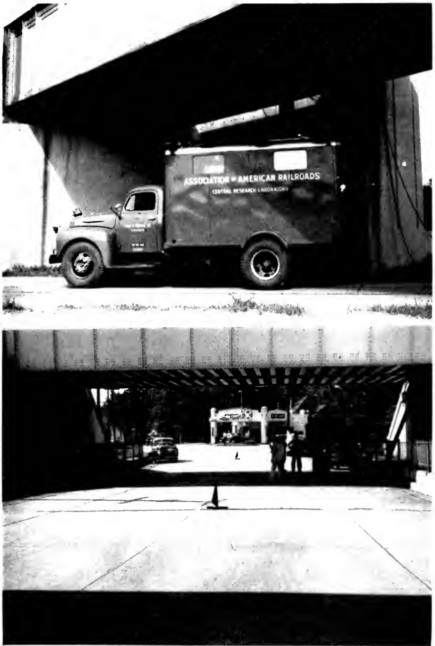
Fig. 3—General views of instrument truck near test bridge.
